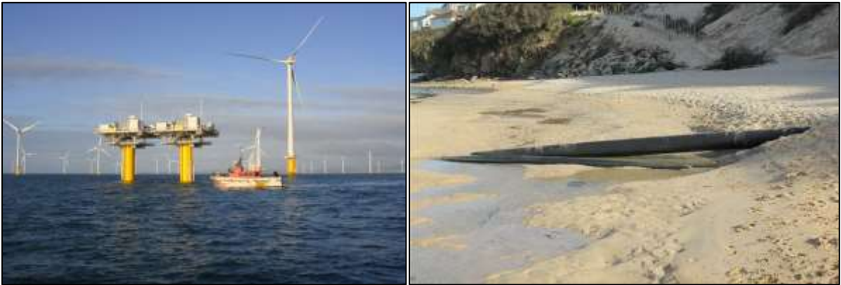
Figure 2 Examples of critical features susceptible to bed level change: offshore wind developments (left) and export cable (right)
